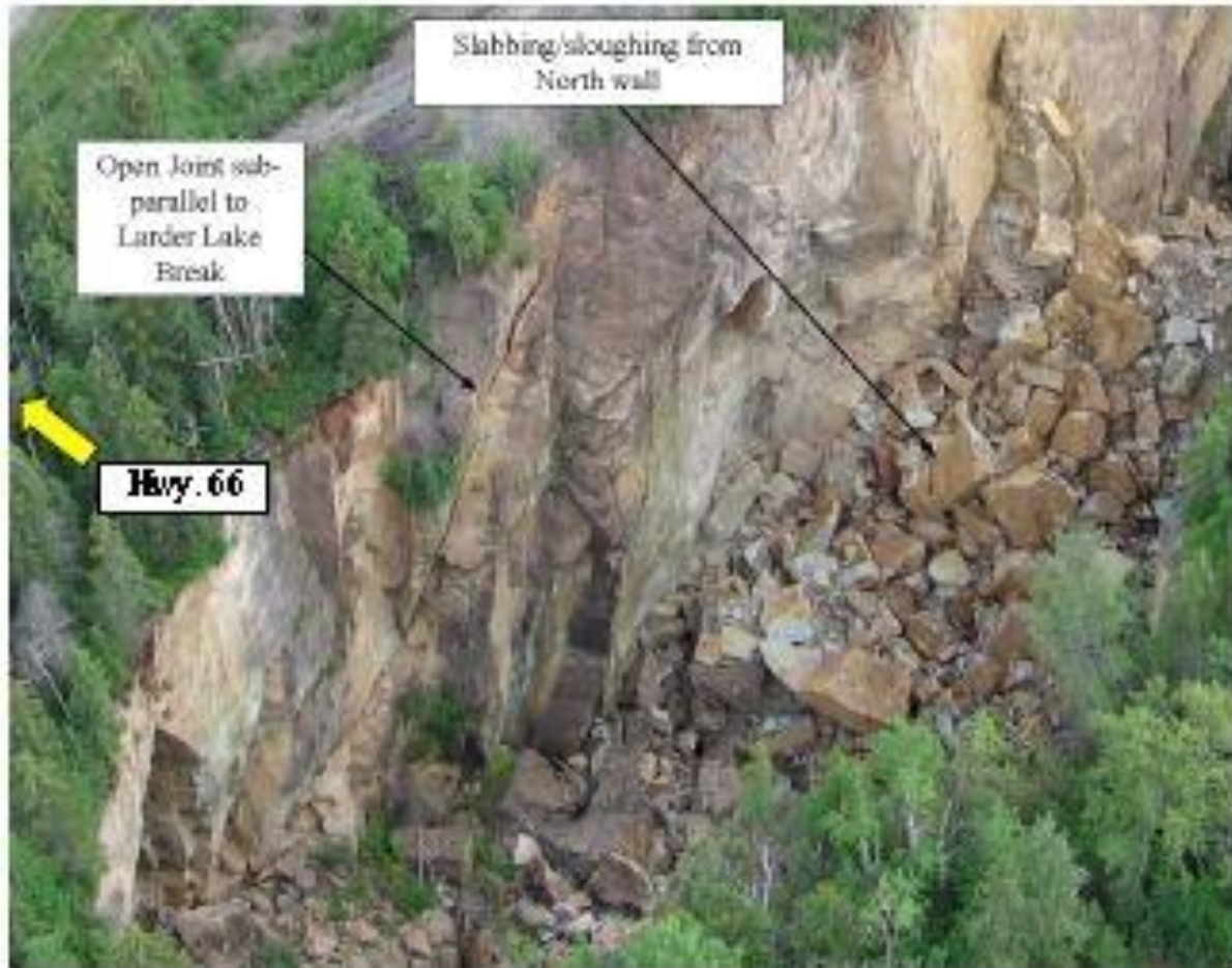
Evidence of on-going progressive hanging wall failure in the West Glory Hole. (ICCI, 2007.)
